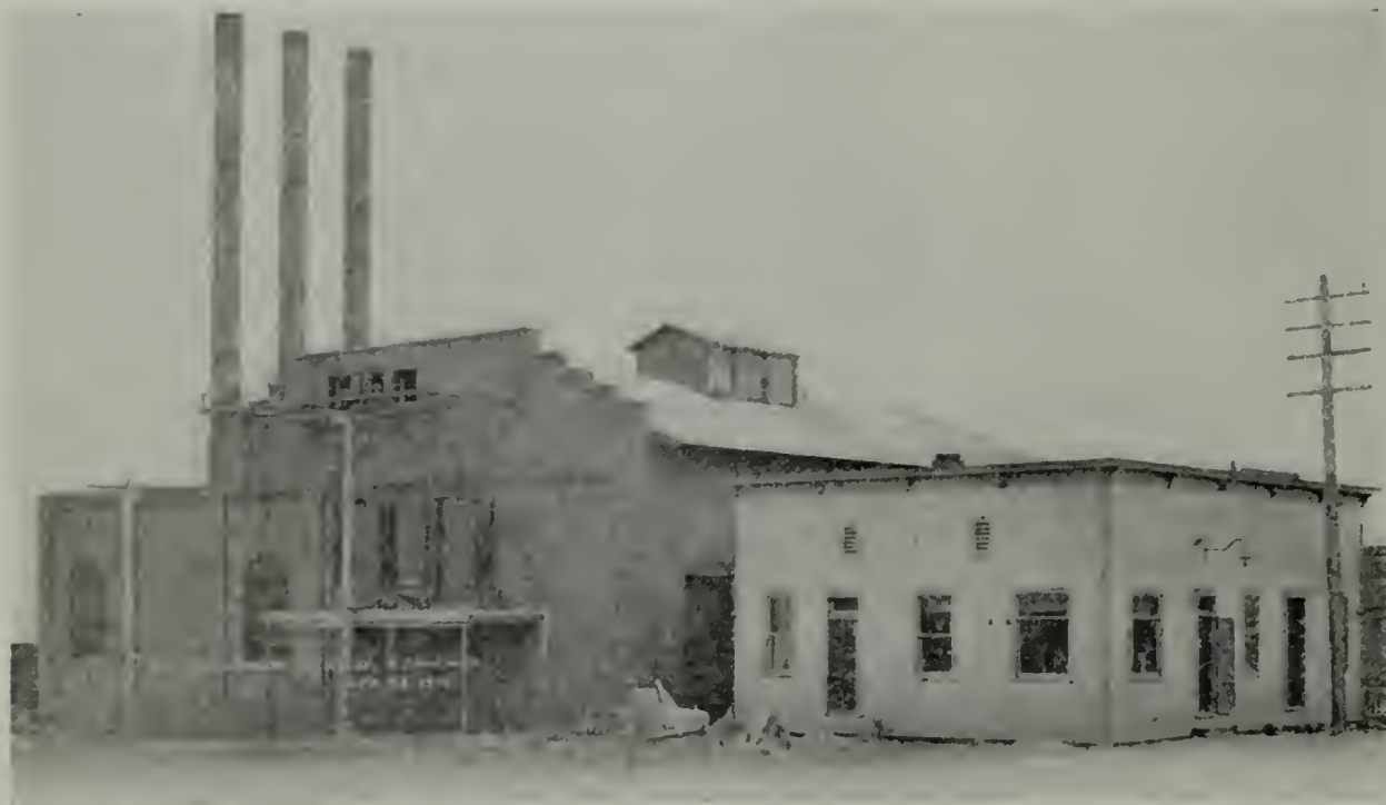
Kennewick Steam Generating Station - July 1, 1910.
